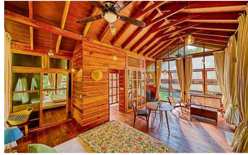
A Kumta-based wooden home designed by Andagere Architects, Gollarapalya, Bengaluru Rural. Interiors of the house have roofing done with marine plywood and coconut timber.
